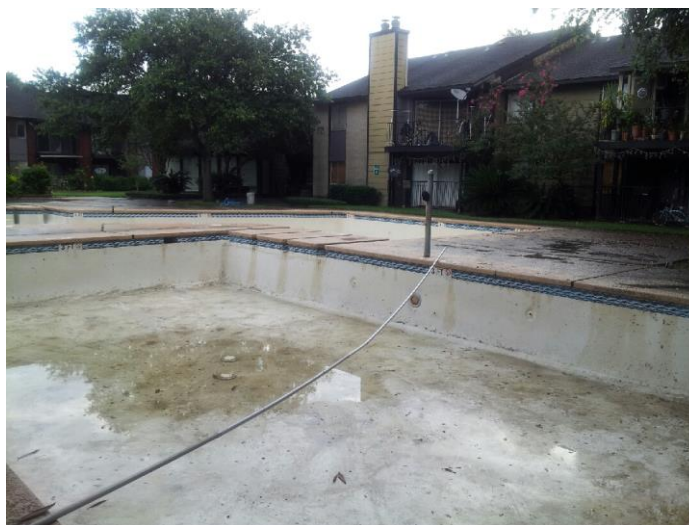
Broken, deserted swimming pool, a serious danger to kids
